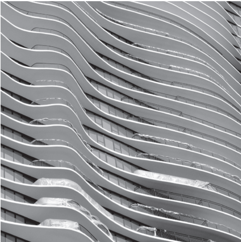
Figure 12.9. Studio Gang's Aqua Tower in Chicago, enclosed only by glass and projecting concrete balconies, acts as an 82-story heat exchanger.
