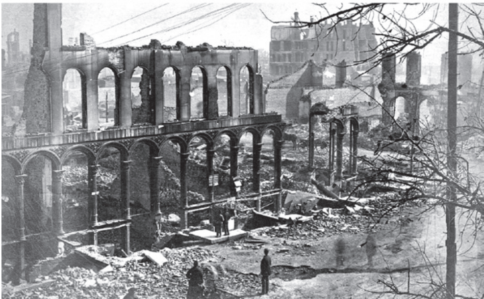
Figure 3.1. The Great Fires of London, 1666 (St. Paul's burning by Wenceslaus Hollar, top ), and Chicago, 1871 (destroyed buildings, photographer unknown, bottom ).
