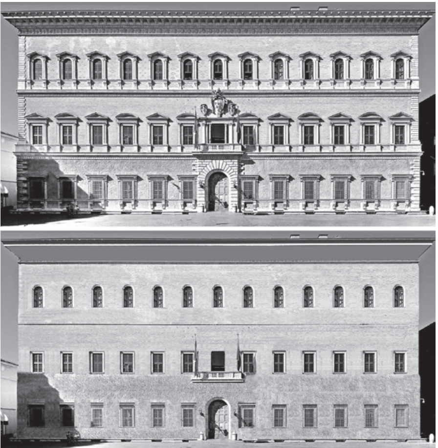
Figure 10.8. The top image shows the Palazzo Farnese, a High Renaissance palace in Rome designed by Antonio da Sangallo the Younger beginning in 1515 (with Michelangelo redesigning the third story and cornice later in the sixteenth century); the bottom image shows the same facade, digitally stripped of its decorative elements.
