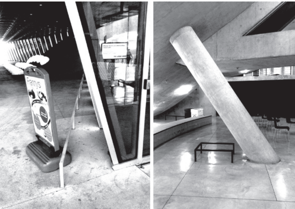
Figure 4.3. Cane detection devices installed at Milstein Hall after the building was occupied, Cornell University, Ithaca, NY.
