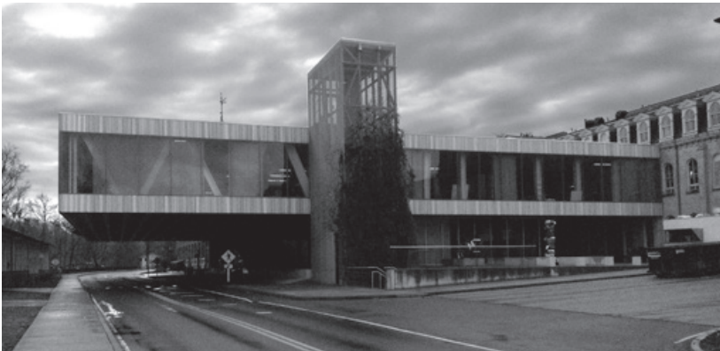
Figure 12.11. Enormous rigid-frame "trusses," visible behind the curtain wall, enable OMA's Milstein Hall at Cornell University (2011) to cantilever over University Avenue.
