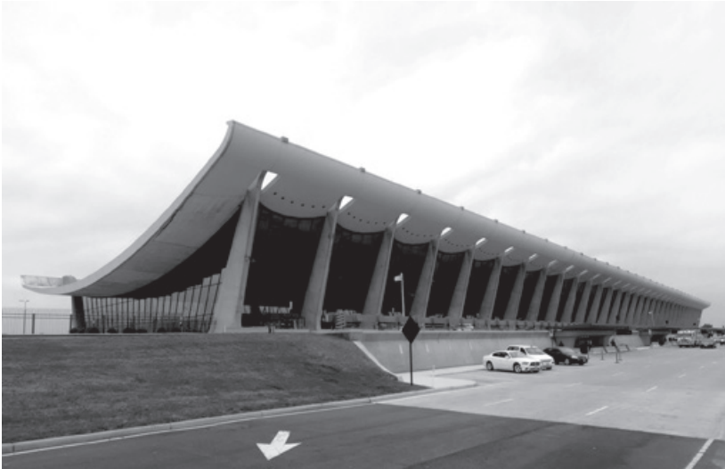
Figure 12.6. Saarinen’s Dulles International Airport Terminal Building: the forms have little to do with structural efficiency but are designed from the point of view of architectural and structural expression.
