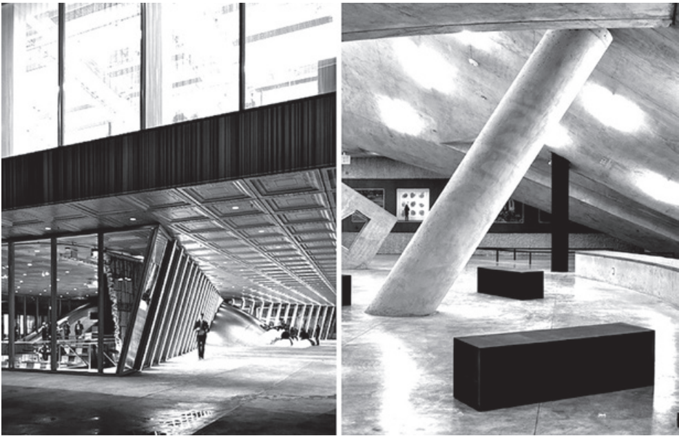
Figure 4.2. Protruding objects in Milstein Hall, Cornell University, Ithaca, NY.
